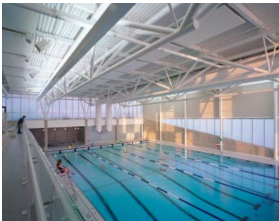
Figure 4: a) Steel roof deck over a steel and concrete structure with perimeter and centralized supply of air; b) Wood deck over a steel structure with perimeter only air supply.
