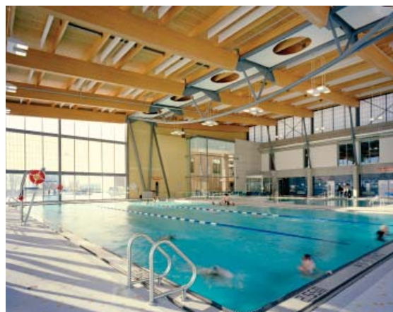
Figure 4: a) Steel roof deck over a steel and concrete structure with perimeter and centralized supply of air; b) Wood deck over a steel structure with perimeter only air supply.
