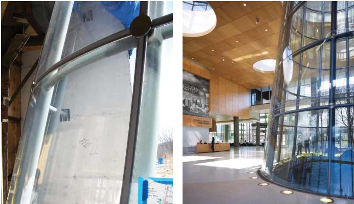
Figure 29: Patch fittings at the corner of glass units (left); Terrarium after construction (right). Photo credit Steve Hall © Hedrich Blessing Photographers.
