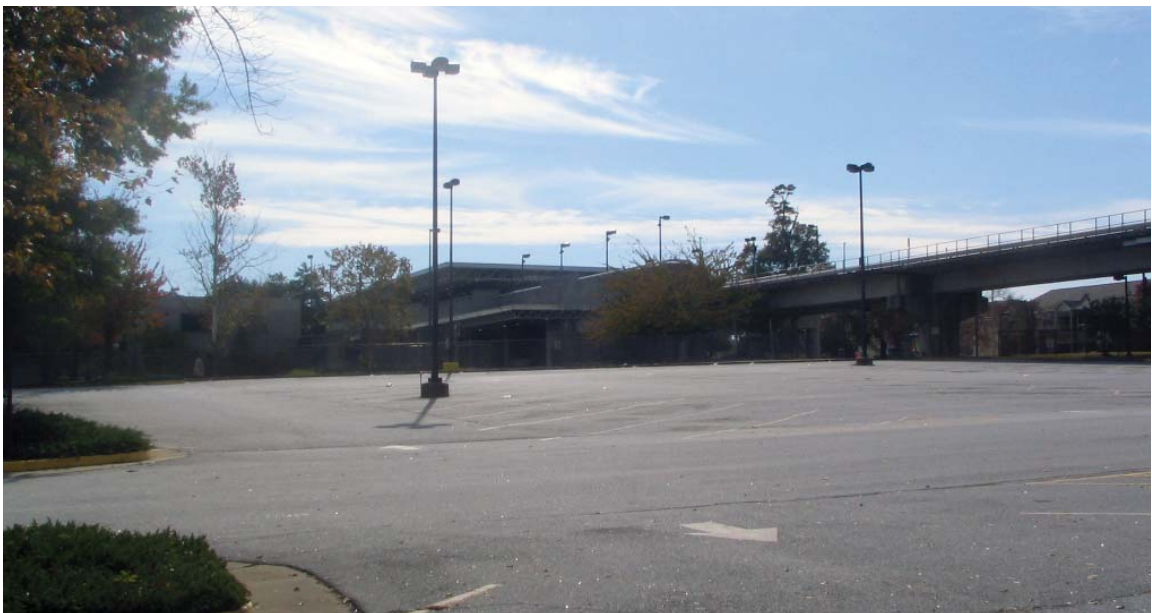
Figure 2: Parking at West End MARTA station (photo: by author).
