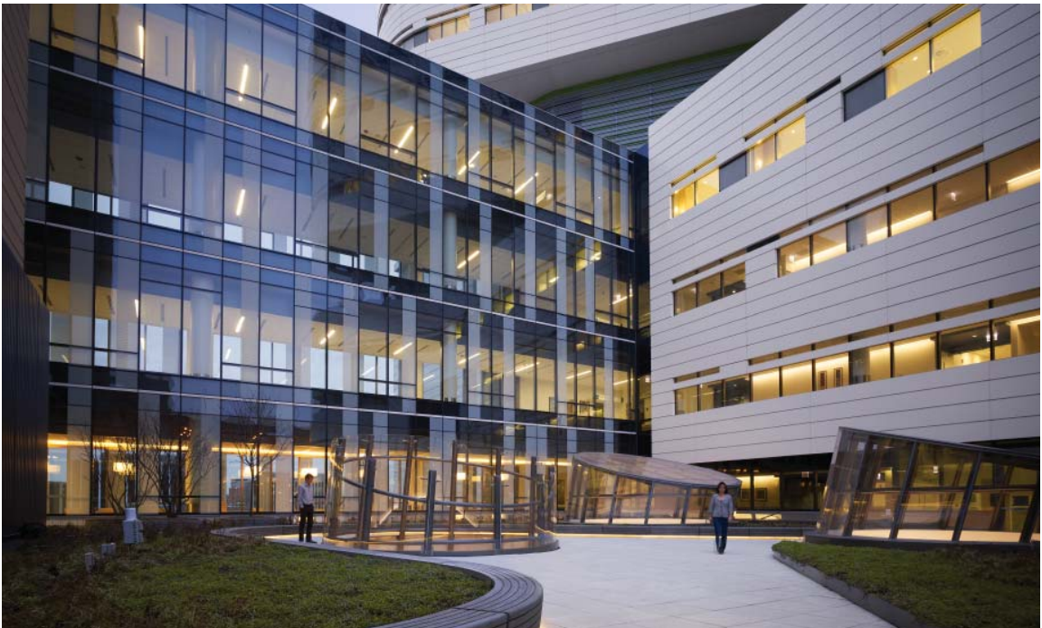
Figure 9: Entry Pavilion roof garden after construction, view from south-west. Photo credit Steve Hall © Hedrich Blessing Photographers.
