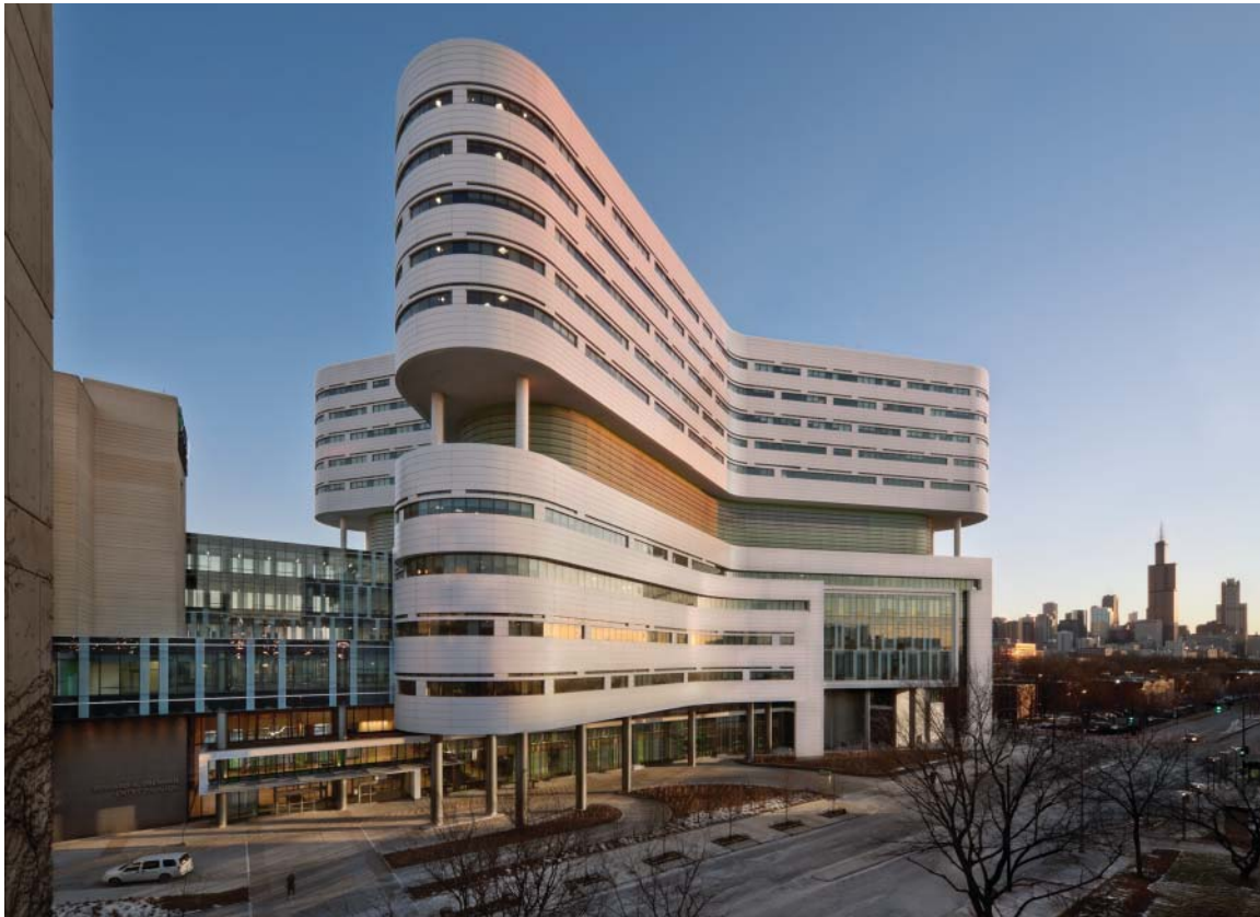
Figure 2: The Tower, view from Harrison Street. Photo credit James Steinkamp © Steinkamp Photography.
