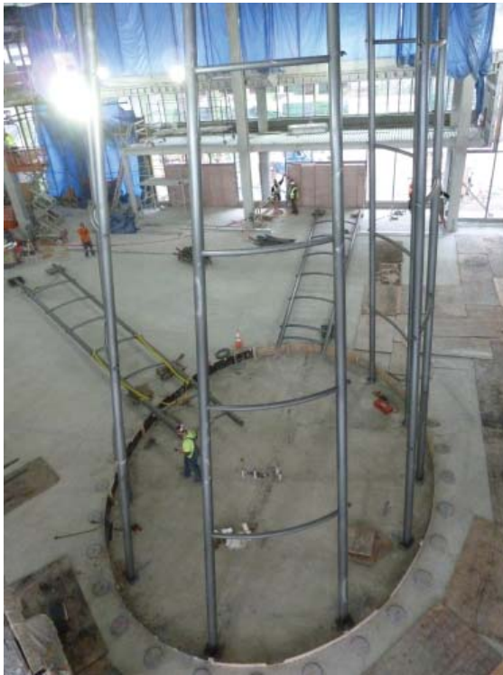
Figure 27: Structural ladders (left); Assembly of the ladders to create the terrarium form (right).
