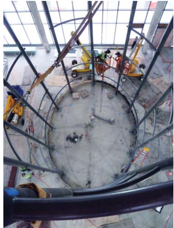
Figure 27: Structural ladders (left); Assembly of the ladders to create the terrarium form (right).
