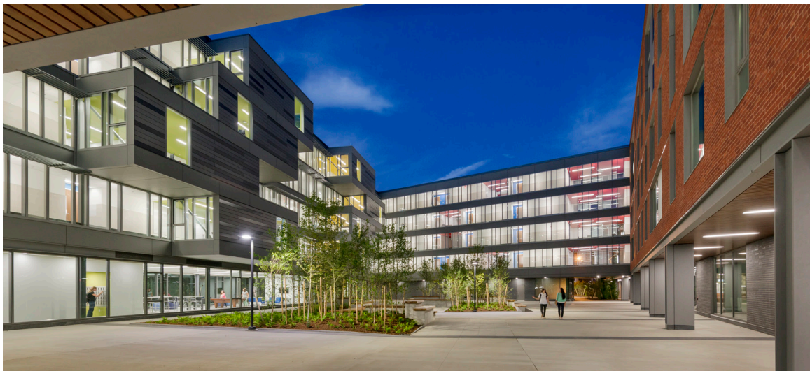
Figure 3: Courtyard at Night—The ground level is open on one side through a loggia that frames a view to the campus lawn. Hundreds of commuting students experience the courtyard on their way to class. At a campus level, this courtyard links to a series of residential green spaces providing students more intimate spaces to retreat and gather as a community.
