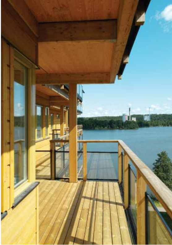
Figure 3: Limnologen (Växjö, Sweden) is supported by local and national programs to expand the timber industry in Sweden. (Photo credit: Midroc Property Development)
