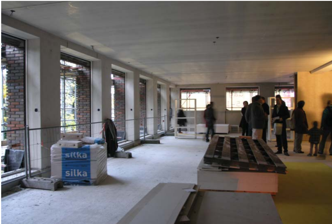
Figure 5: Interior of Solid Oud West under construction.
