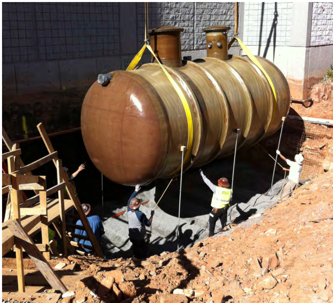
Figure 7c: 10,000-gallon cistern under construction.
