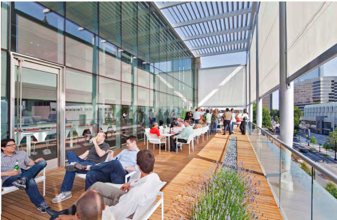
Figure 6d: A steel trellis and motorized shade system prevent solar heat gain and glare from the west. Photo credit Eduard Hueber © Arch Photo, Inc..
