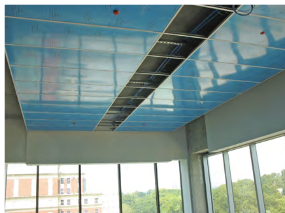
Figure 4: Radiant heating and cooling system (water-filled blue BEKA mats above suspended ceiling tiles).
