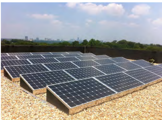
Figure 5: a) Heat recovery unit, also referred to as an “enthalpy wheel”. b) Raised floor system with underfloor air distribution. c) 7.2 kW Photovoltaic array on roof.
