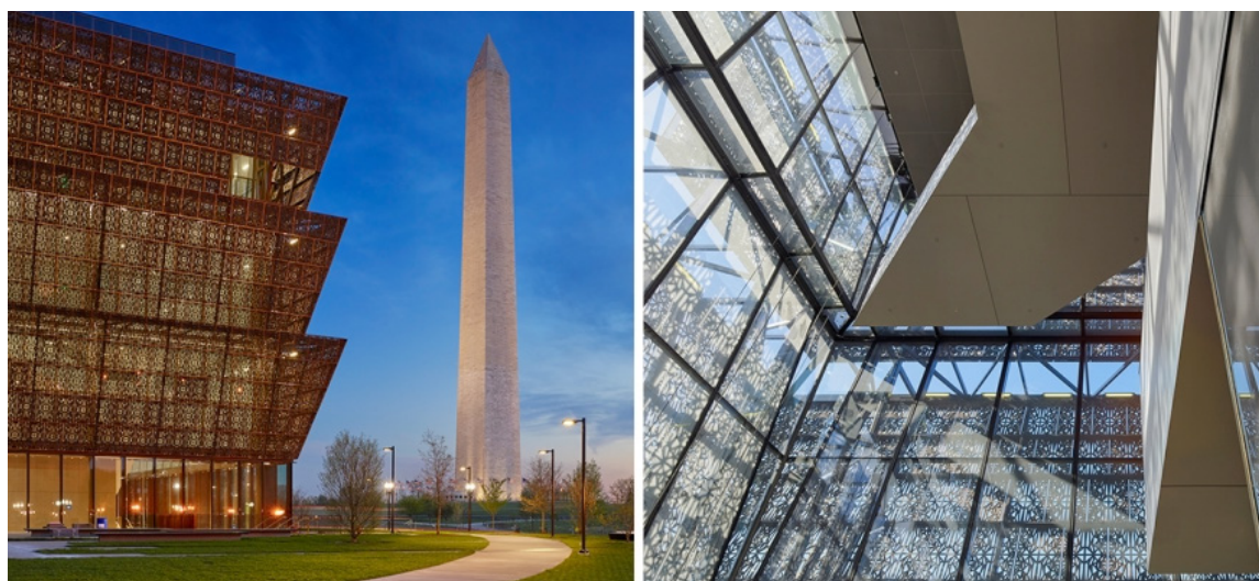
Figure 6: External shading through a screen defines the form of the NMAAHC. This application balances views and solar performance.
