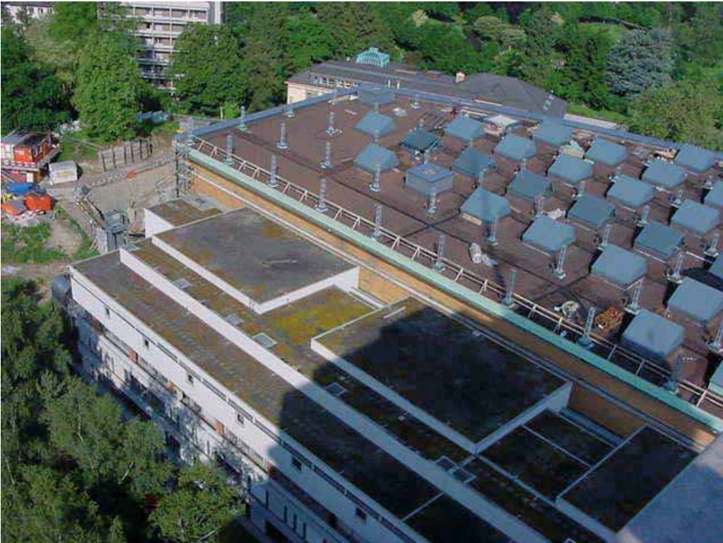
Figure 6 Roof of Phase One of Primary System - a “green” roof with skylights
