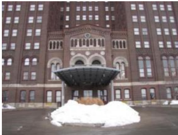
Figure 5.18: Site B - View of Main Entrance
