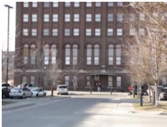
Figure 5.30: Site B – View of Two Story Windows from Exterior
