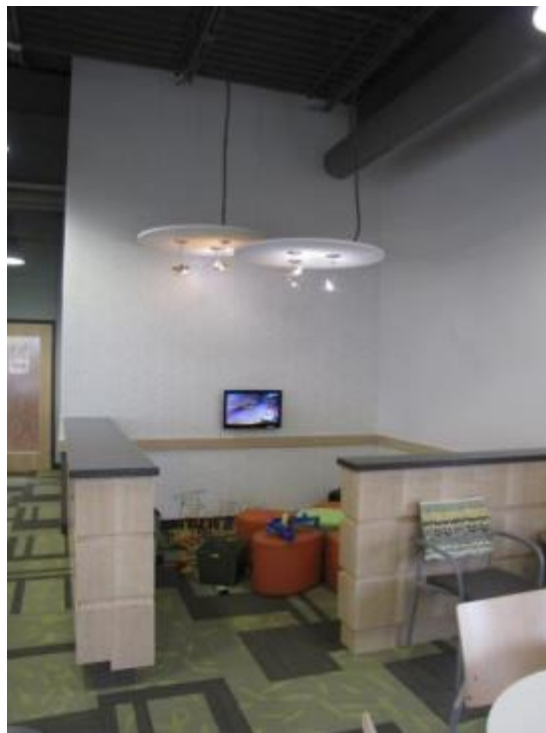
Figure 5.9: Site A – View of Suspended Ceiling in Children's Play Area
