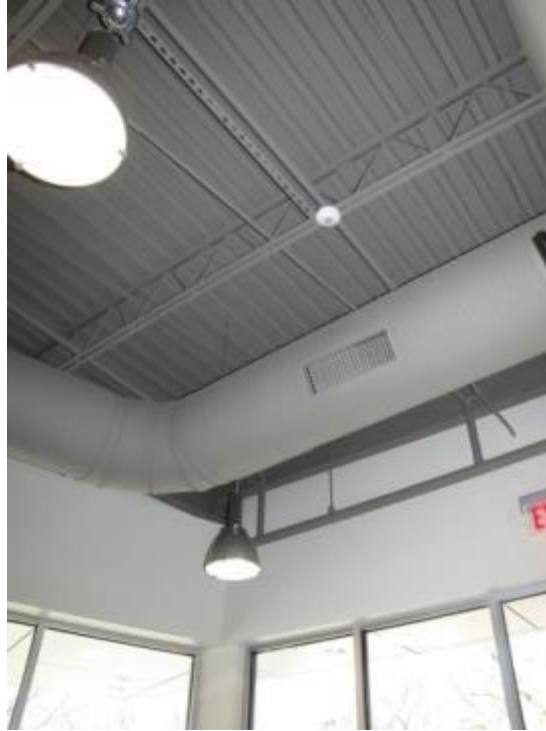
Figure 5.8: Site A – View of Exposed Ceiling
