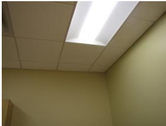
Figure 5.16: Site A – View of Acoustic Ceiling Panels
