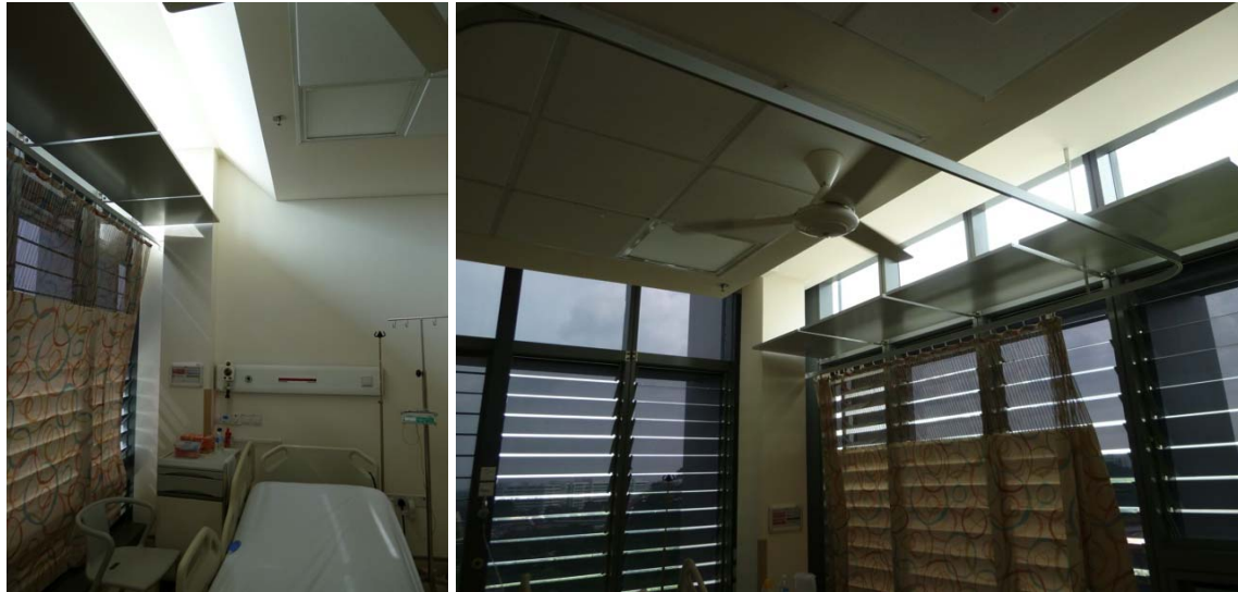
Figure 3-21 Sub-performing shading devices/light shelves
