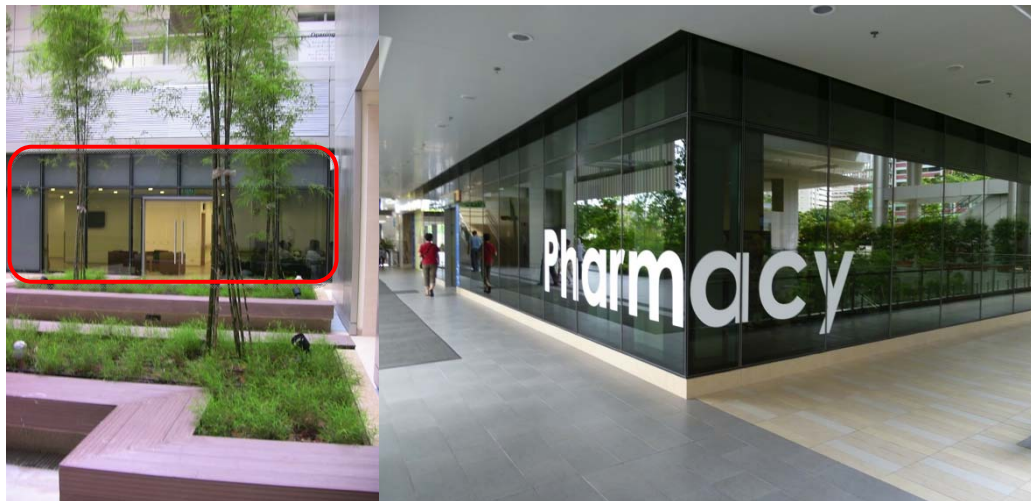
Figure 3-19 Inappropriate use of window treatments (Left: Low-e glass used for façade in basement of hospital (as highlighted in red); Right: tinted windows for pharmacy)
