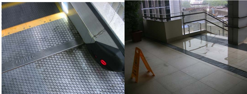
Figure 3-13 Rain-exposed vertical transportation (Left: Escalator showing rainwater seepage; Right: staircase showing flooded area)
