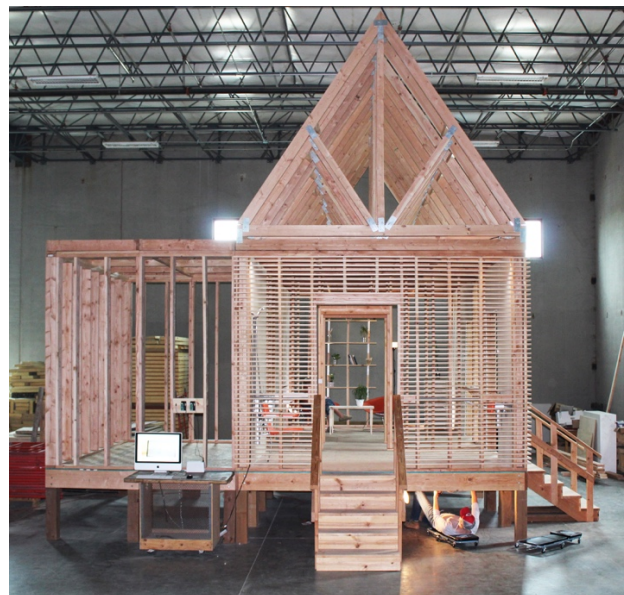
Fig. 8. Smart Home mock-up construction, Institute for Smart Cities, University of Kansas
