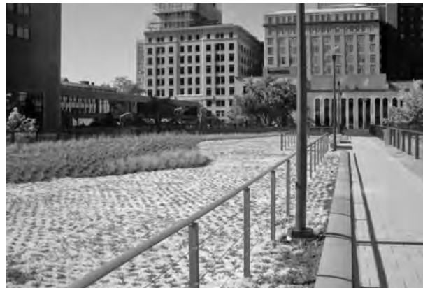
▲ After renovation of plaza to a green roof system.
