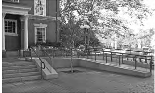
▲ Code-compliant accessibility features, like ramps and handrails, can be added to historic plazas without compromising aesthetics.
