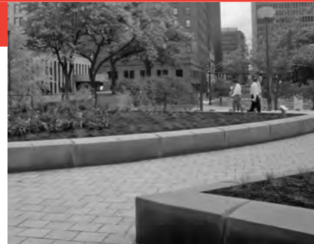
▲ Wide, faceted joints and grooves in sitting walls prevent skateboarding along the edge.
