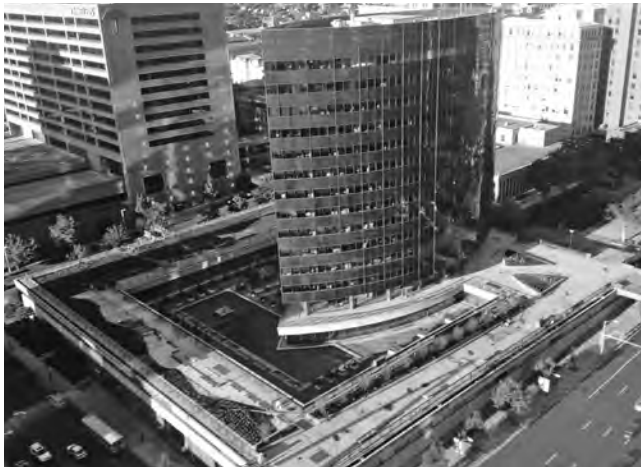
▲ A plaza project offers the opportunity to enhance the stature of a property and raise its value to the community.
