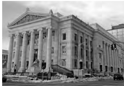
▲ New Haven Courthouse in New Haven, Connecticut. Marble Facade Restoration.
