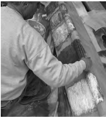
▲ Mockup test of stripping agents to remove prior inappropriate coating.
