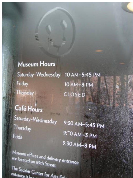
Fig. 4: Condensation at exterior glazed enclosure. (2005) © Angel Ayón, WASA/Studio A.
