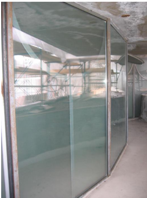
Fig. 5: New IG unit on steel- frame in front of original glazed enclosure. (2007) © Angel Ayón, WASA/Studio A.
