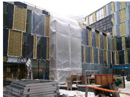
Figure 34: Temporary exterior heating via test specimen.
