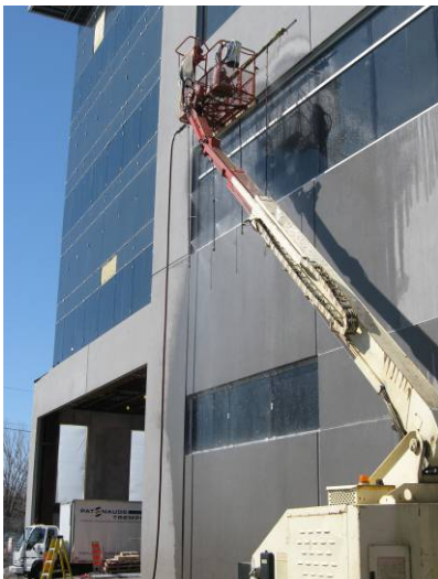
Figure 12: Field testing for resistance to water penetration.
