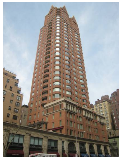
Figure 4: Aluminum punch windows and brick cladding (New York, NY)
