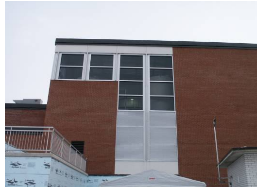
Figure 36: Diagnostic hose testing window/wall interface.
