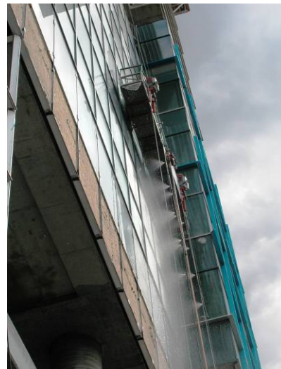
Figure 13: Field testing for resistance to water penetration.
