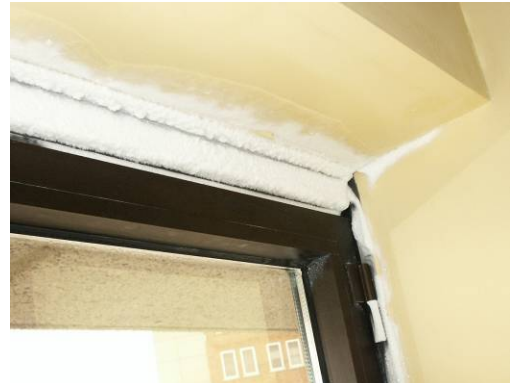
Figure 8: Example of excessive interior frost formation due to excessive air infiltration at a window/wall interface.
