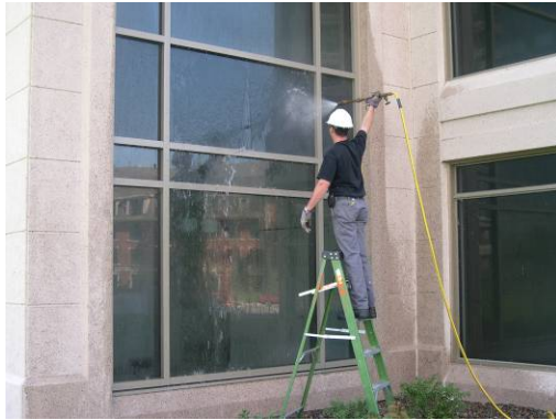
Figure 35: Diagnostic hose testing of curtain wall section.
