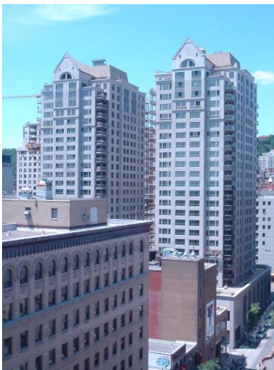
Figure 3: Aluminum punch windows and precast concrete (Montreal, QC)
