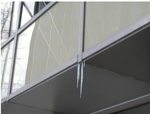
Figure 7: Example of exterior icicle formation due to excessive air exfiltration within a curtain wall assembly.
