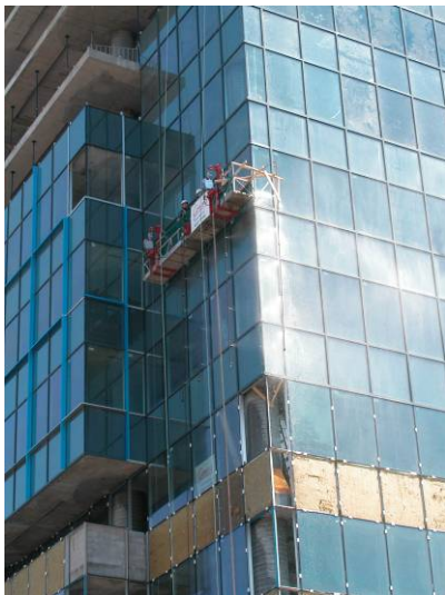
Figure 31: Calibrated sprinkler rack hung from suspended scaffolding.
