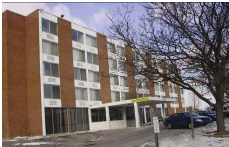
Great Lakes Rehabilitation Hospital before renovation Photo: Contracting Resources
