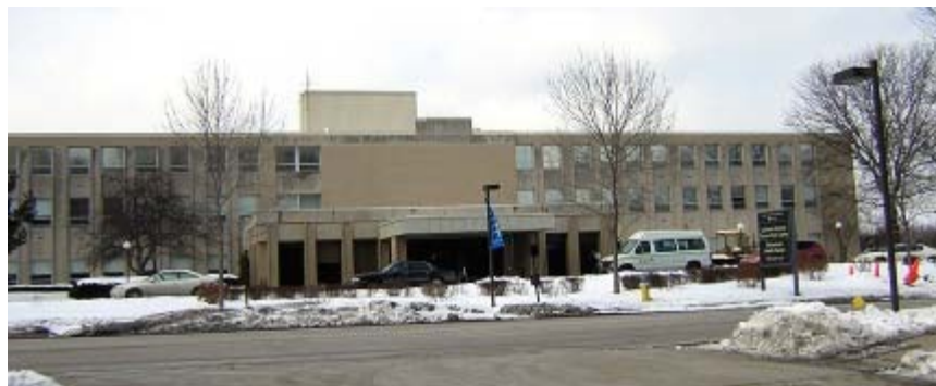
Image 2. ALGH existing facade Photo: OWP/P
