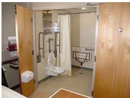
Image 4. "Bathroom with double-leaf door to accommodate easy access for patients" Courtesy of author.
