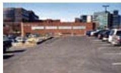
Figure 4: The existing radiation oncology service's understated two-story brick structure with no sense of entry may easily be mistaken for a campus maintenance building.
