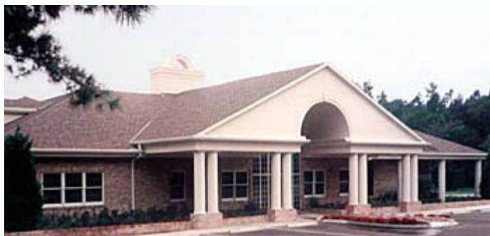
Figure 1: The exterior of the Ocala Radiation Therapy Center projects a residential accented vocabulary with its mansard roofs, deep overhangs, and chimney. the 16-foot high concrete vaults are in effect screened with residential materials.
