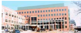
Construction Photo - Cancer Institute of New Jersey
