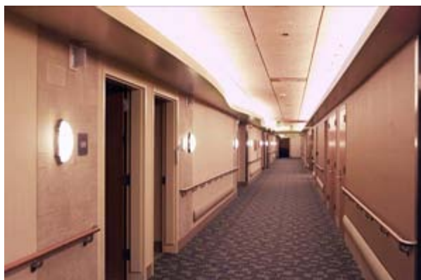
Indirect lighting in a corridor is more soothing to a patient lying on a gurney. 4
