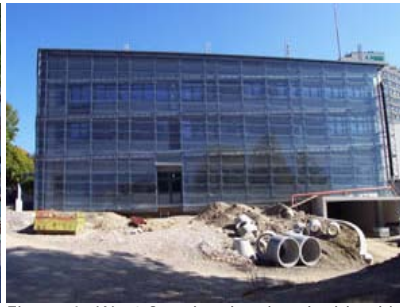
Figure 6: West façade, showing double skin
