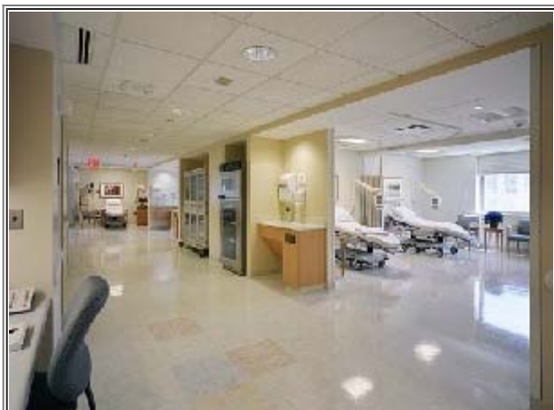
Photo courtesy of KMD Architects The Post-Anesthesia Care Unit is broken into clusters containing two beds each, creating a sense of privacy for patients while still allowing good sightlines for nurse supervision.
