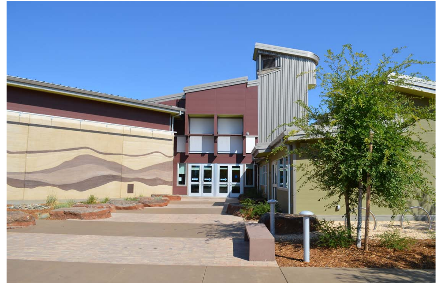
Image 1: The entry to Redding School of the Arts showcases the traditional building method of rammed earth walls. The materials and vegetation along with path complement the natural surroundings of the site.
