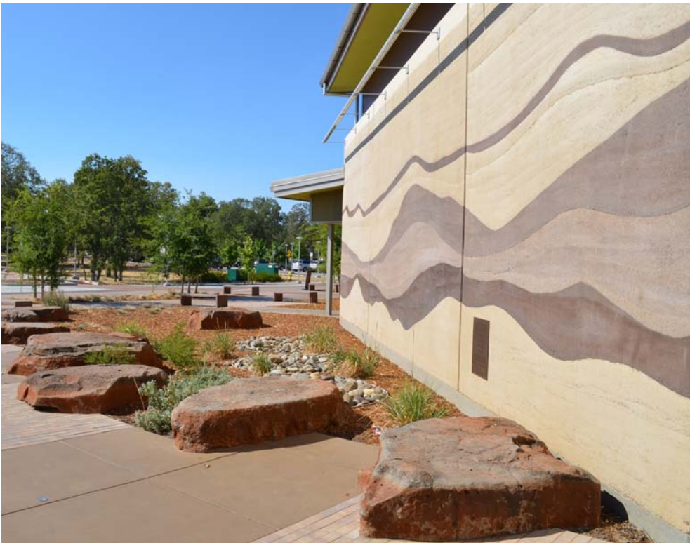
Image 3: The 24” rammed earth wall provides insulation from the sun for the music and dance rooms on the other side of the wall.
