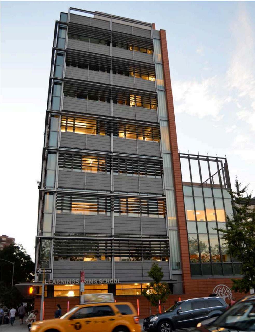
Image 3: The custom exterior shading system provides light and thermal comfort for LearningSpring School.
