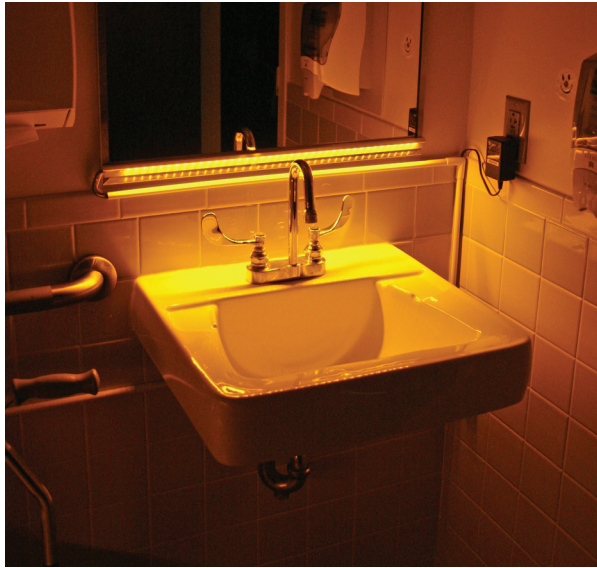
Figure 2a and 2b. Motion-sensor controlled amber LEDs installed at sink (left) and toilet (right) areas.
