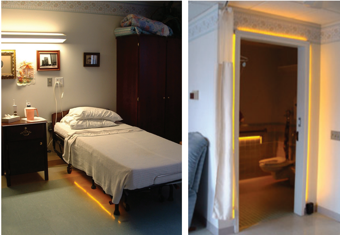
Figure 1a and 1b. Motion-sensor controlled amber LEDs installed under bed (left) and around doorway (right). Notes: 1) photosensors were disconnected for the photos; 2) overhead fluorescent luminaire was kept off after installation of night-lighting.
