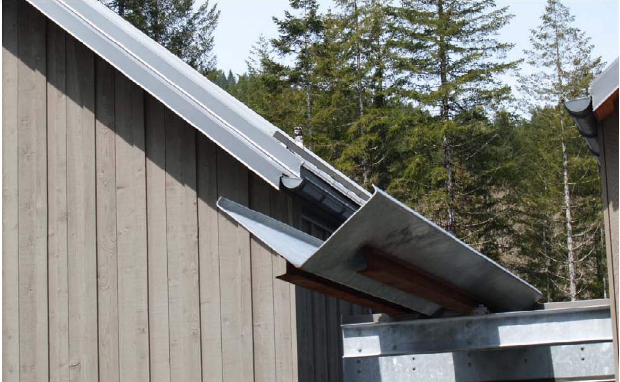
Fig. 3. The scupper that collects rainwater between the two roof planes and delivers it to the pond
