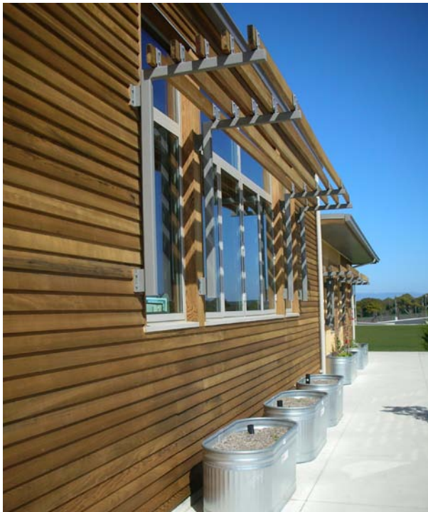
Fig. 9. Southern shading system and recycled wine-cask siding
