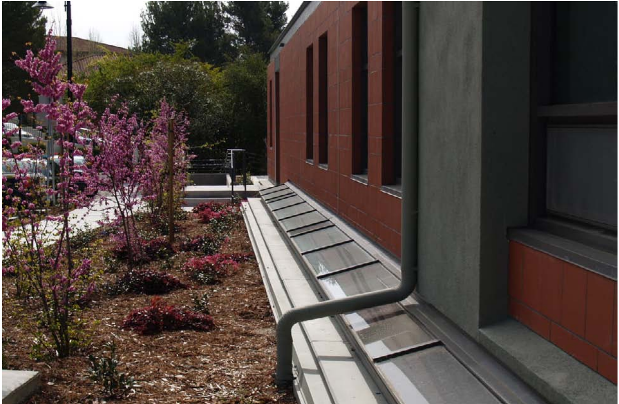
Fig. 13. Detail of the skylights to the lower level
