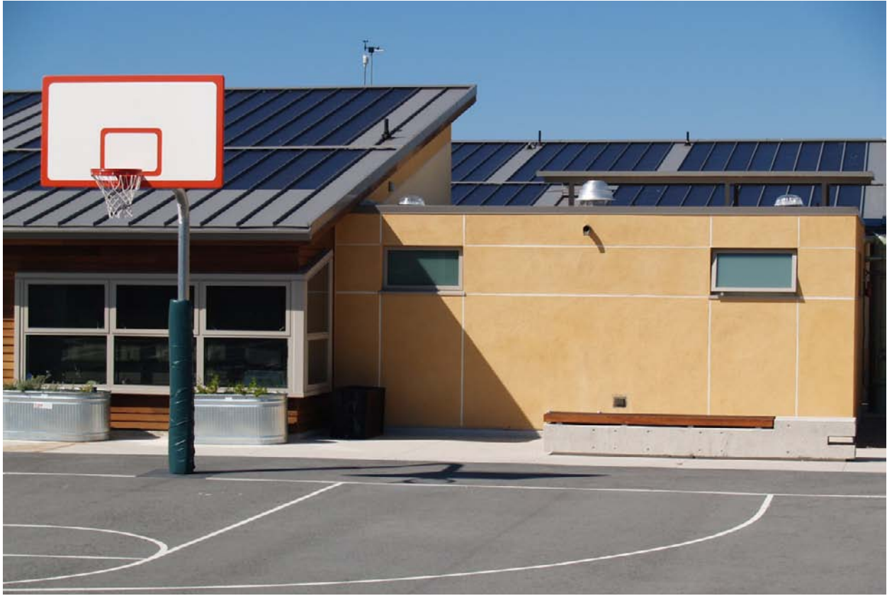
Fig. 8. Integrated roof-mounted photovoltaic panels
