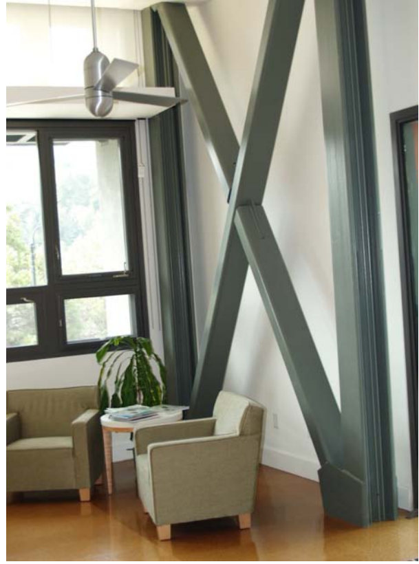
Fig. 16. Interior character and cross-bracing
