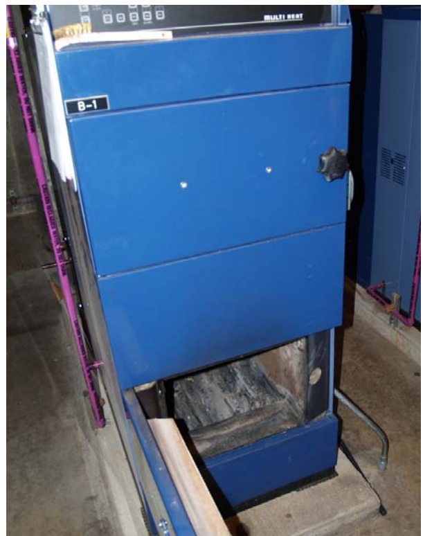
Fig. 10. The pellet boiler in the mechanical room
