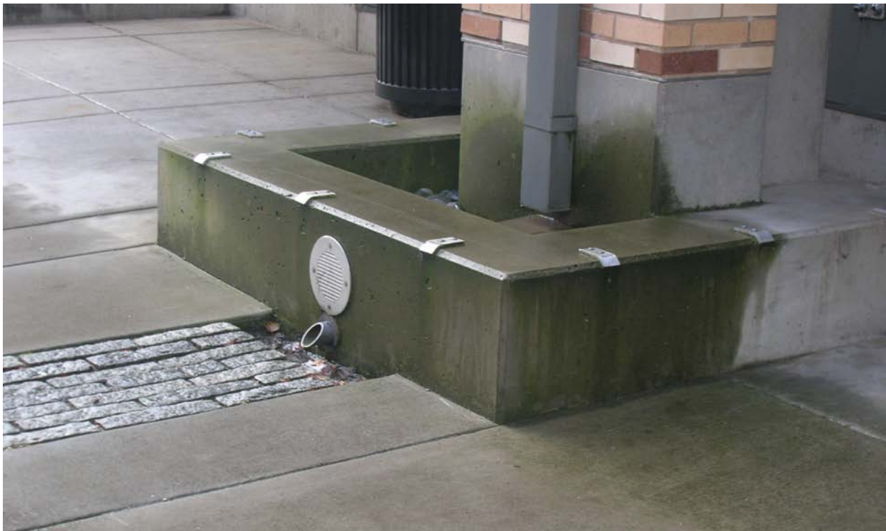
Fig. 6. Detail of the downspout system and its connection to the runnel across the alley
