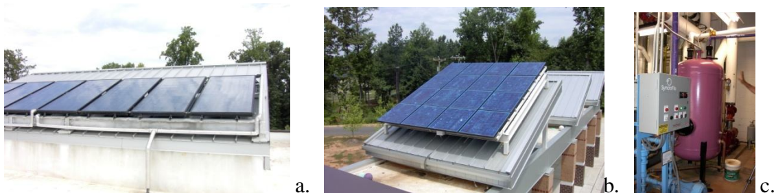
Figure 2. a) Thermal solar water heating system, b) photovoltaic array, and c) rainwater filtering system.
