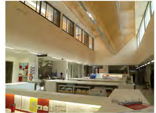
Figure 117: High clerestories in Intensive Care Unit for effective daylight penetration, Alfred Hospital, Melbourne, Australia.
