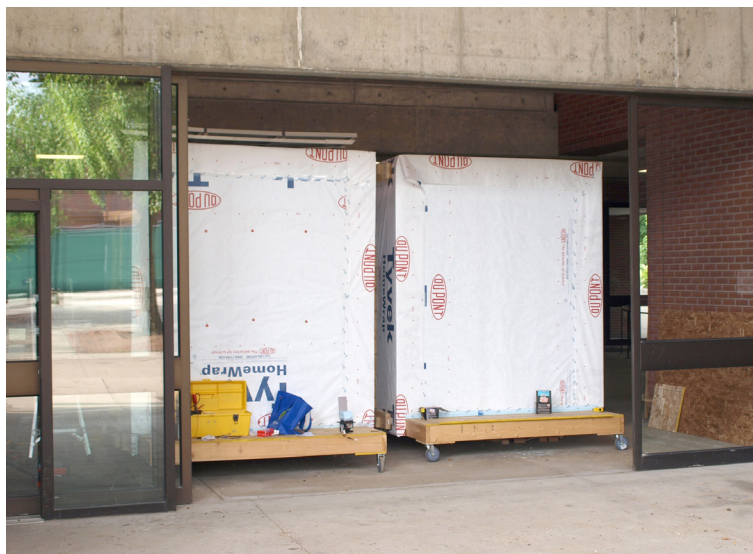
Figure 1: The two prototypes being moved to an exterior roof deck.
