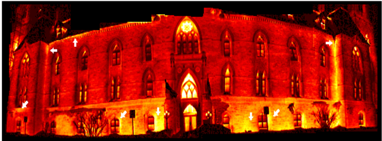
Figure 11. Ground floor of solid masonry wall assembly illustrates warmer surface temperatures due to rising damp from ground water in foundation wall.
