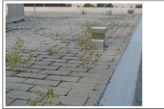
Figure 4. Visual of concrete clad insulation over inverted roof membrane, no visible wetting on concrete.
