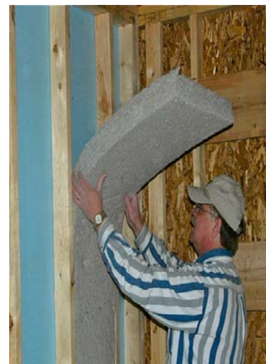
Figure 4: Installation of cellulose batt
