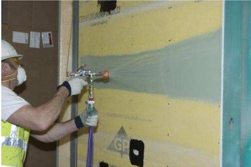
**Figure 7:** Treatment of gypsum sheathing joints per air barrier assembly.
