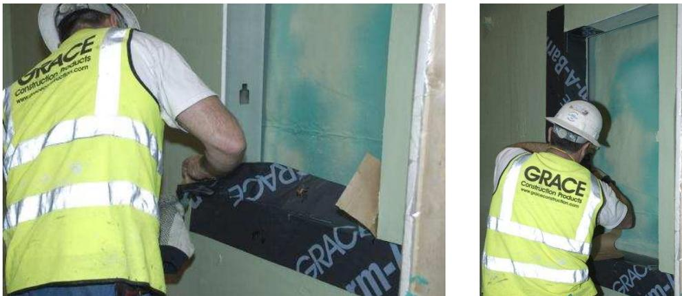
**Figure 8:** Flashing windows with a fully adhered membrane.
