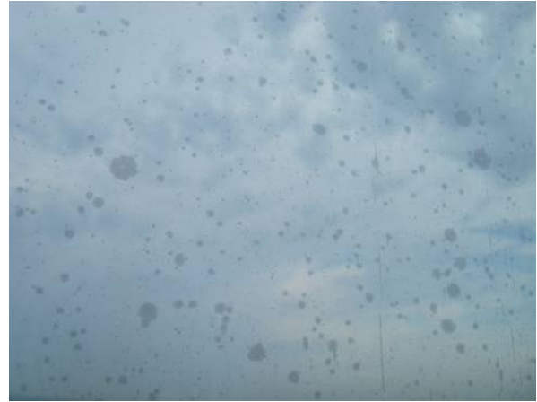
Figure 8: Large spots within the insulated glazing units
