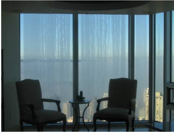
Figure 7: Visual condensation and severe corrosion of the low-e coating visible from the interior
