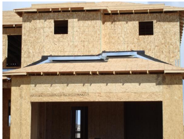
Figure 2: Continuous sheathing
