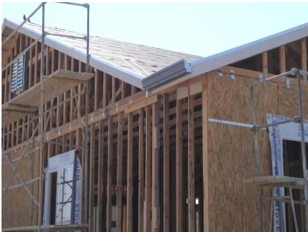
Figure 1: Sheathing only at shear locations
