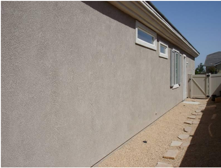
Figure 7: Wall area that required control joints
