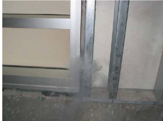
Figure 1: ASTM E 1186 Smoke Tracer Test at a mock up to locate air leakage locations
