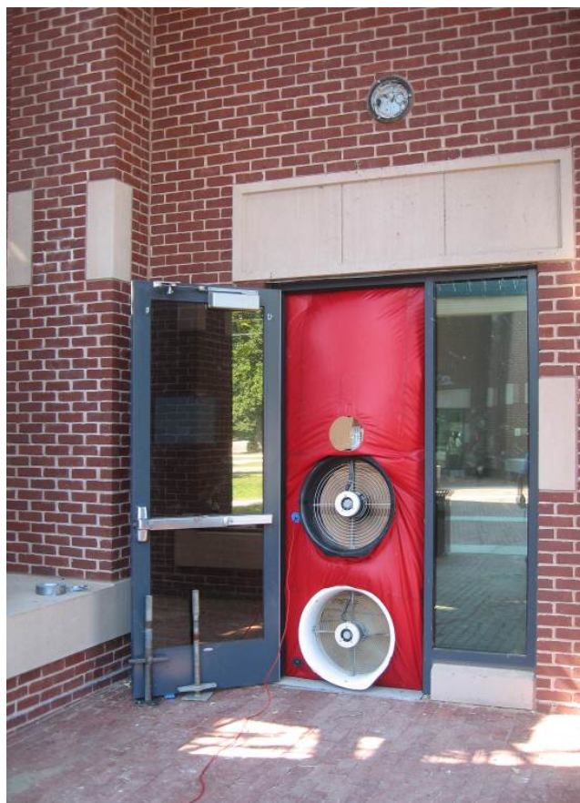
Photo 9 – Test setup for blower door test with calibrated fans.
