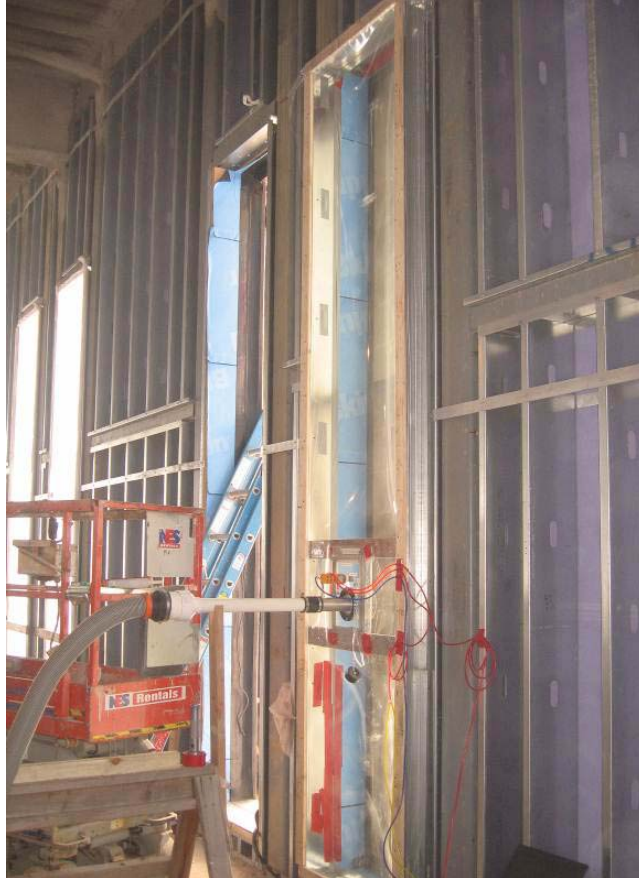
Photo 6 – Air leakage testing for an air barrier-to-fenestration transition on a building.
