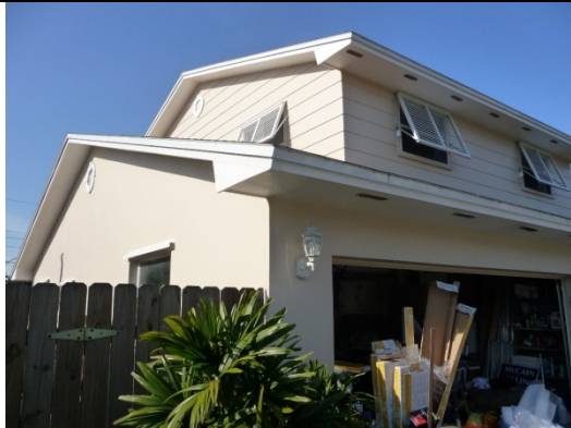
Figure 12 Shallow attic at front of house H11C. Oval vents allow air from outside into attic. No peak or off-peak vents were used.
