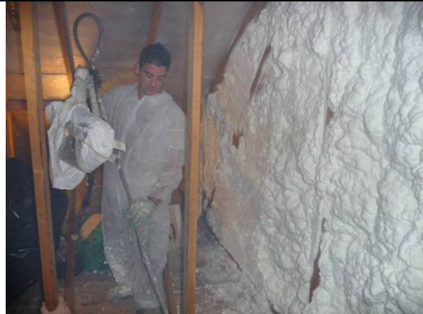
Figure 8 Technician finishes up kneewall and floor cavity insulation/air tightening. (Ian LaHiff)
