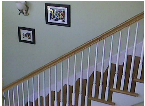
Figure 3 Visual image of stairwell. The location of the floor cavity can be referenced to the location of the pictures. (Withers)
