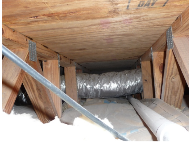
Figure 19 View inside floor cavity taken from opening to attic space. (Withers)
