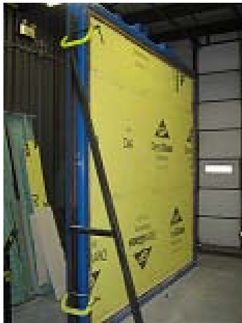
Figure 2: Base wall prior to installation of foam plastic insulation
