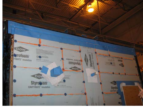
Figure 10: Completed wall with penetrations sealed
