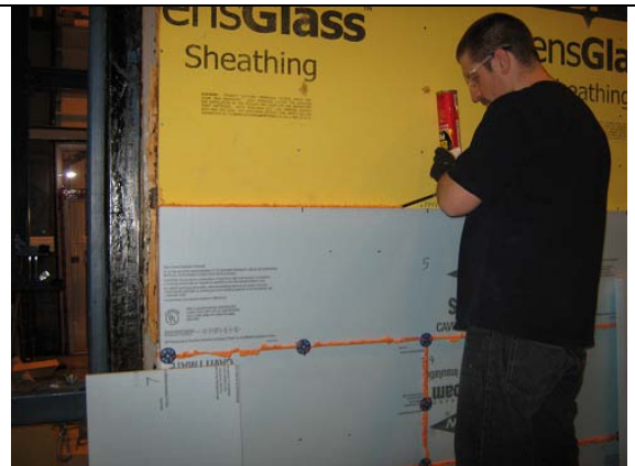
Figure 8: Installation of XPS and foam sealant
