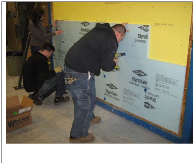
Figure 3: Installing the XPS insulation
