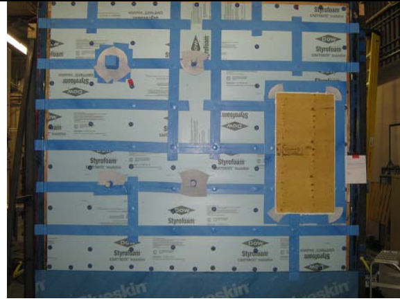
Figure 6: Completed wall with sealed penetrations
