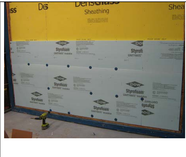
Figure 4: Several XPS boards installed
