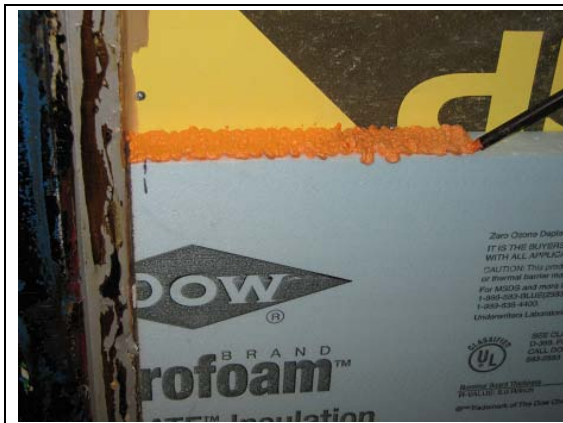
Figure 7: Foam sealant applied to edge
