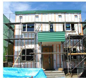
b) External Insulation Technique
