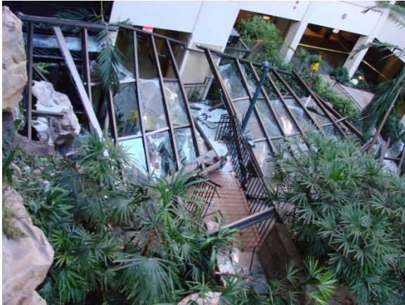
Figure 10 Sloped glazing built in 1980's investigated after collapse. 2008 Performance
