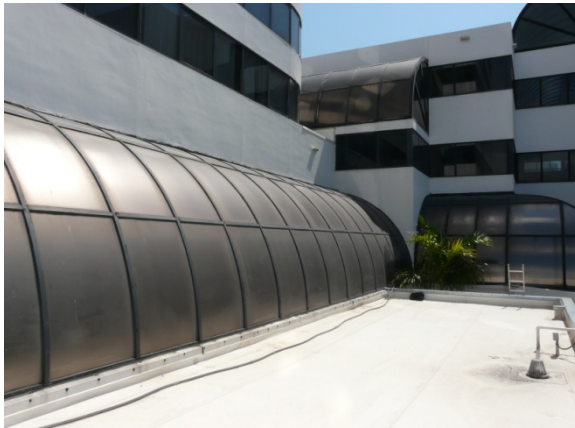
Figure 18 Popular (bad) example of the eave discharge below the sill flashing and roofing, causing the leak in the food court below. West Palm Beach, FL.
