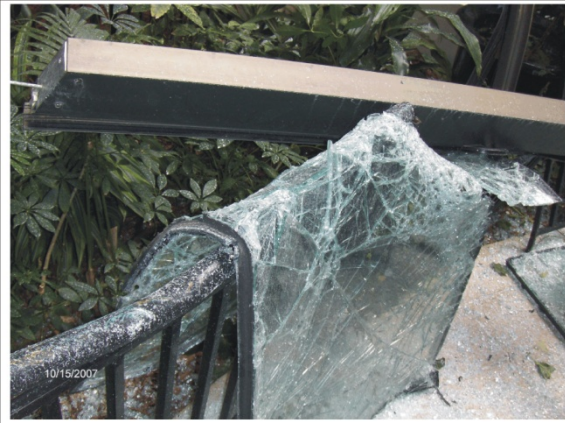
Figure 20 Collapse of the sloped glazing due to thrust inadequately resisted by anchor points.
