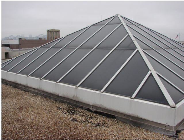
Figure 6 One of typical pyramid-shaped skylights built from 1950's in Gretna, LA.
