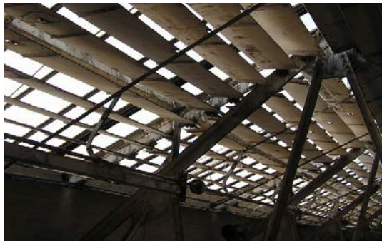
Figure 4 Operable internal louvers in 1916 skylight.
