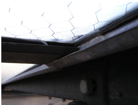
Figure 3 Condensate drainage in 1916 skylight in Cleveland Museum of Art, Cleveland, OH.
