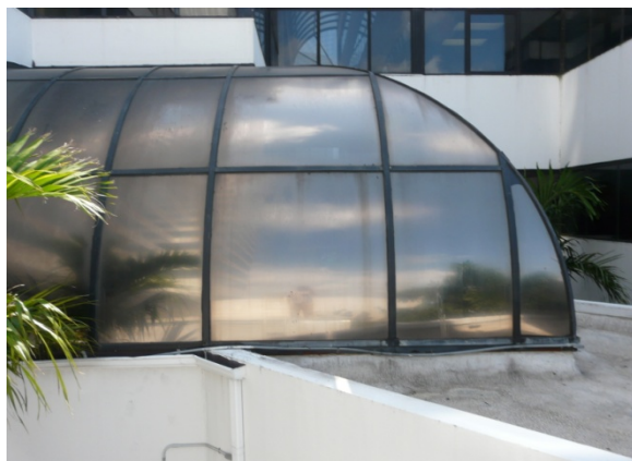
Figure 28 Corrosion and exterior condensation on pyrolytic coating. West Palm beach, FL 2011.
