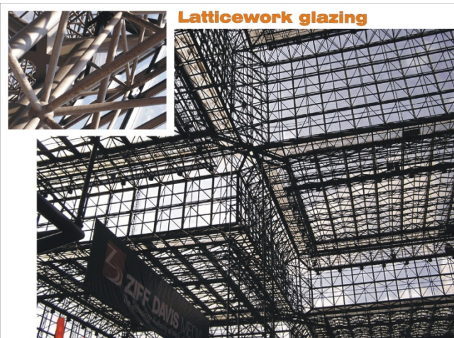
Figure 7 Sloped glazing on a latticework in Jacob K. Javits Convention Center in New York City in 1980's.
