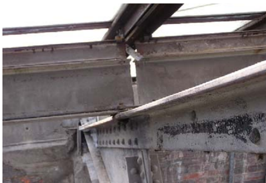
Figure 5 Movement joint with split rafter in the 1916 skylight.
