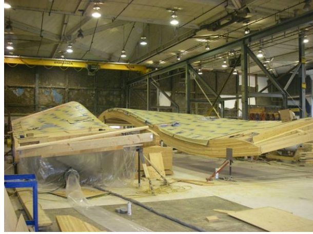
FIGURE 5: Individual Panels Protected with Membrane
