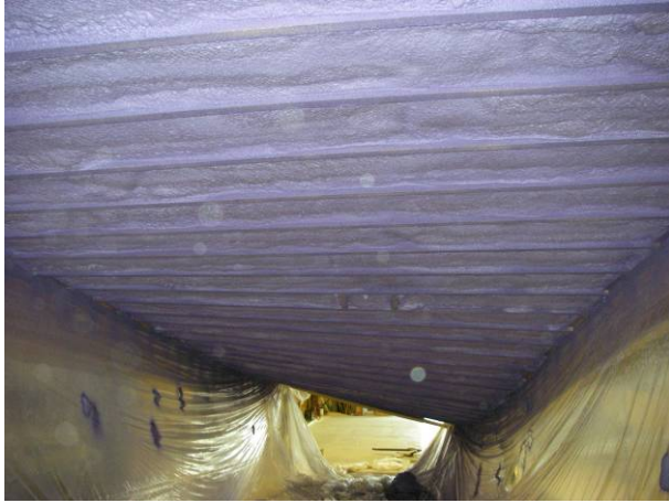
FIGURE 4: Spray Polyurethane Foam Insulation Applied to Underside of Panels
