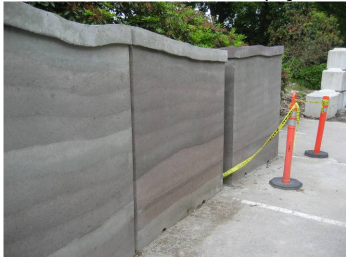
FIGURE 7: Rammed Earth Wall Mock-Up
