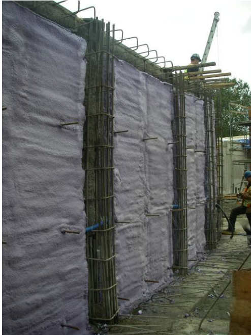
FIGURE 6: Installation of Rammed Earth Sandwich Wall Assembly
