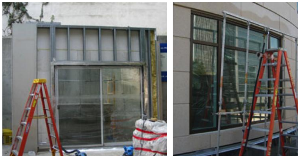
Figure 5. Field mockups are built on-site and differ in whether it is a pre-installation or a first in-place installation: a) Left image shows a “pre-installation” field mockup built adjacent to the building and b) Right image shows a field mockup which is “in-place” meaning that it is installed on the building and if approved will be a permanent installation.
