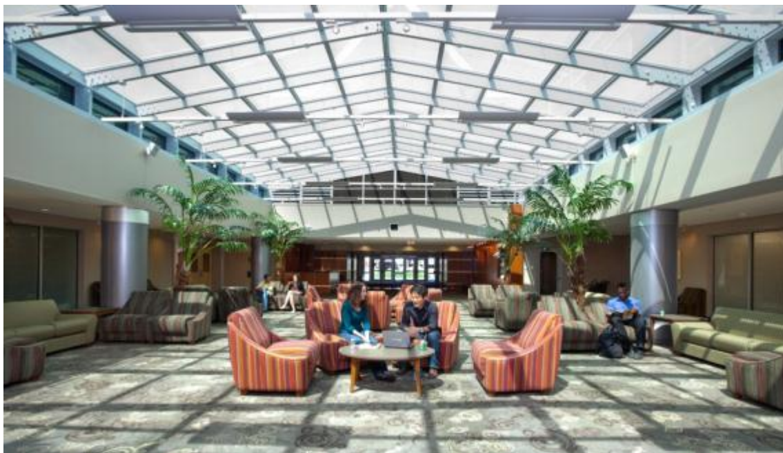
FIGURE 8: Dehority Hall at Ball State University. A fully EC glazed roof with clerestory encloses a courtyard to provide a multiuse space. This image shows the EC glass in the clear state condition with the clerestory in the fully tinted state.
