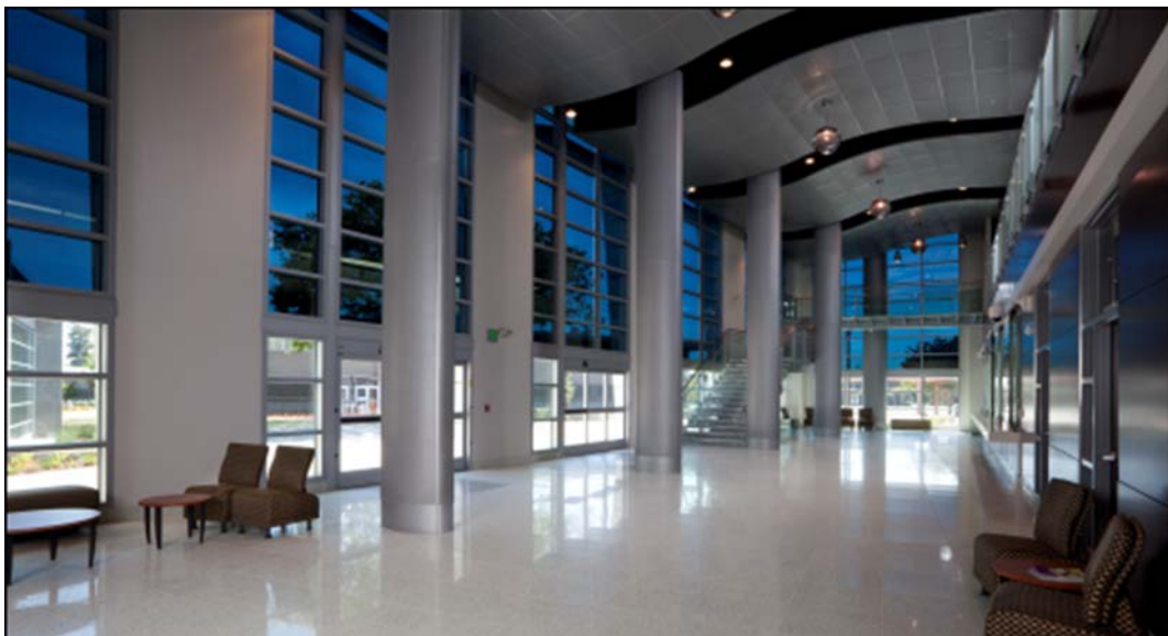
FIGURE 4: Interior view of the EC glass installed in the Student Services Center at Chabot College, Hayward, CA. The glass can be tinted to control the amount of solar heat entering the space to allow effective use of the natural ventilation system.
