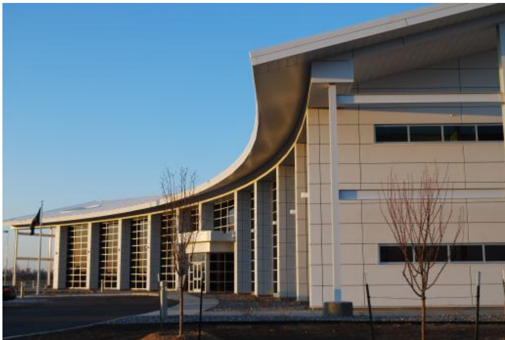
Figure 12: Siemens Wind Turbine Facility, Hutchinson, Kansas. The façade design features EC glass for a clean aesthetic, instead of a horizontal mechanical louver system.
