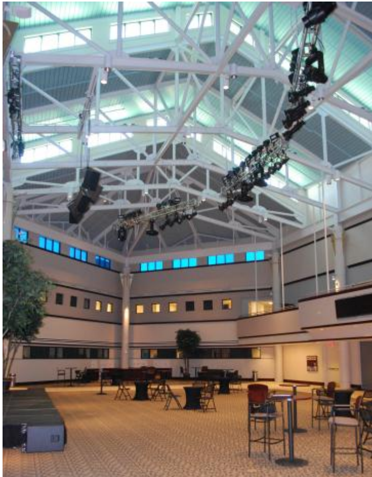
FIGURE 11: Immanuel Bible Church, Springfield, Virginia. EC glass is installed in all the clerestory glazing. In this image, the clerestory at the far end is tinted (the panes on the left hand side are tinted more than those on the right hand side), and the panes in the two tiered clerestories in the foreground are in the fully clear state.
