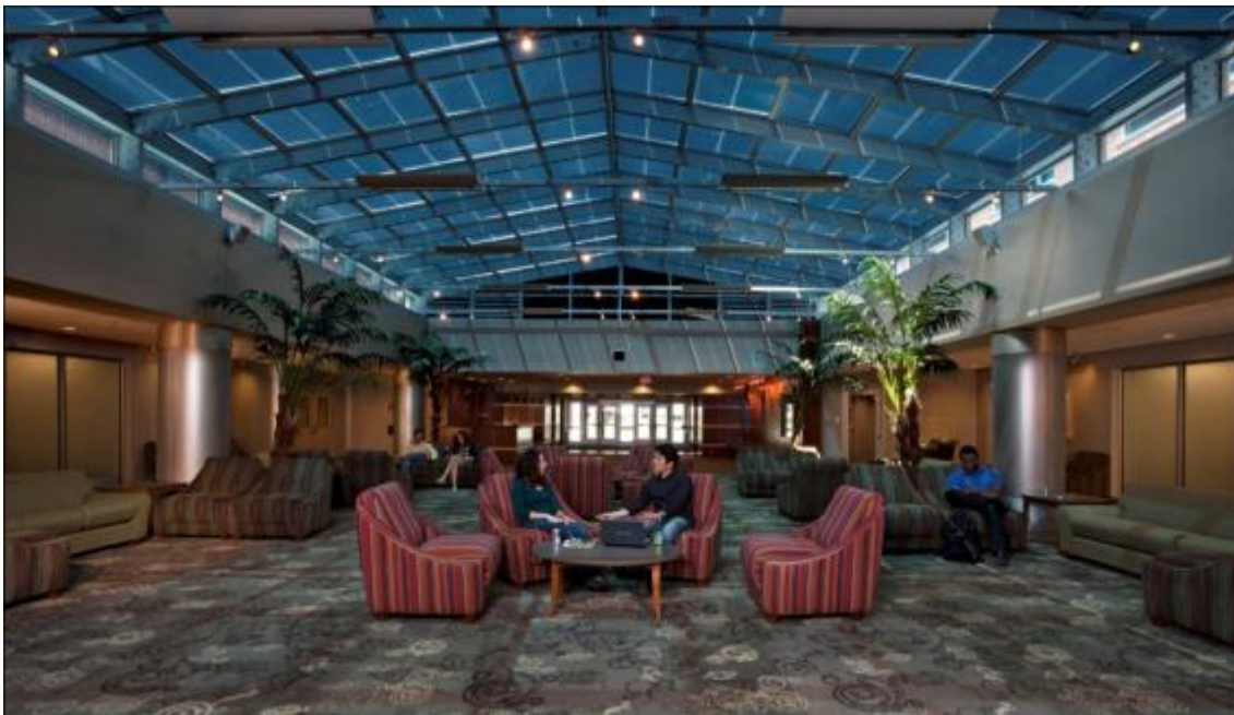
FIGURE 10: Dehority Hall at Ball State University. In this image, the glass is in the fully tinted state ready to provide the necessary light control for AV presentations.
