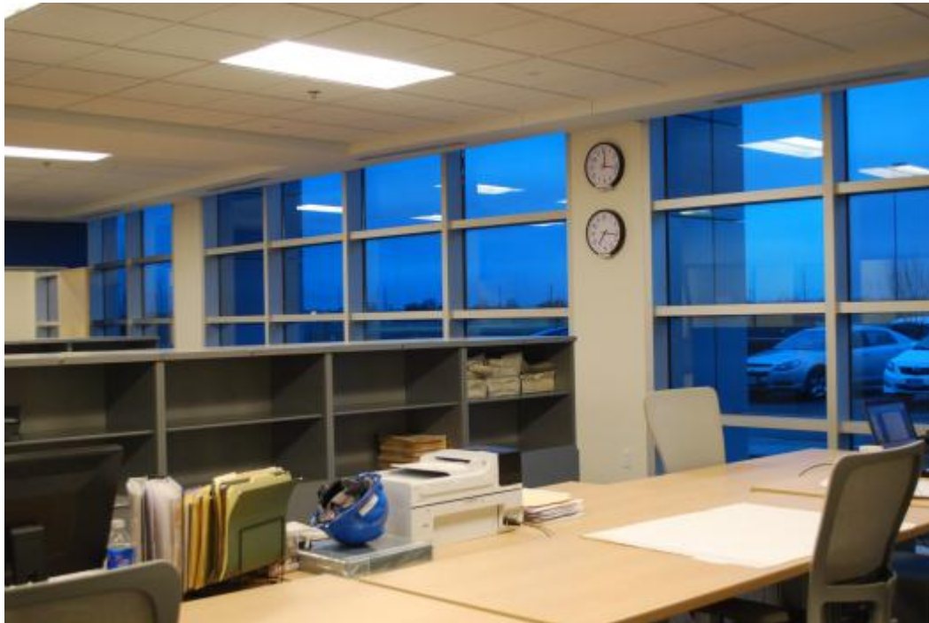
FIGURE 13: View from the inside of the Siemens Wind Turbine Facility. The EC façade encloses private and open office space (shown here) as well as communal areas such as the cafeteria in which AV presentations are given during the day utilizing the light dimming capability of EC in lieu of blinds.
