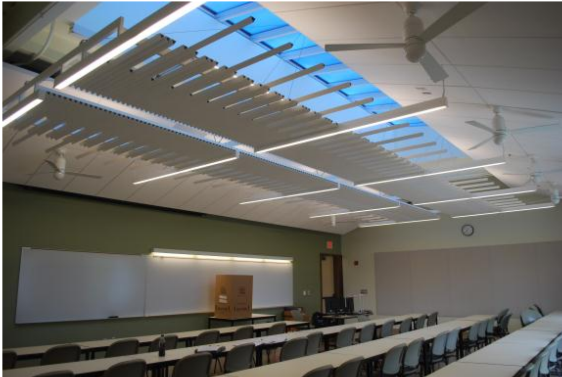
FIGURE 7: An interior view of one of the skylights with EC glass with the light diffuser underneath in a classroom in the Chemeketa Health Science Center. The use of light redirecting techniques in combination with EC glass allows uniform natural daylight penetration into the building while dynamically controlling for heat and glare.
