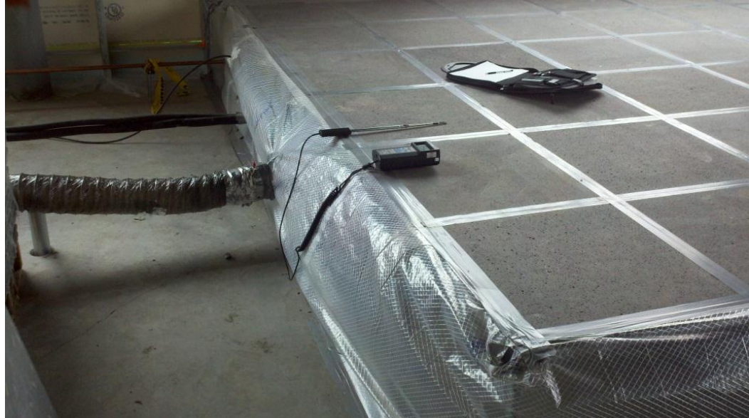
Figure 6 - Access Floor Mockup Pressure Test
