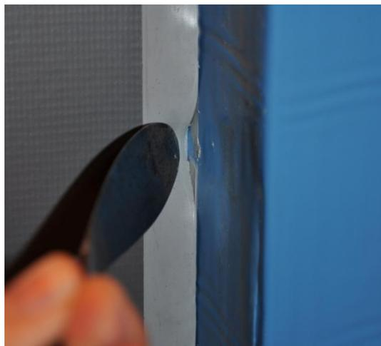
Figure 10. Traditional sealant losing adhesion to the SAF.
