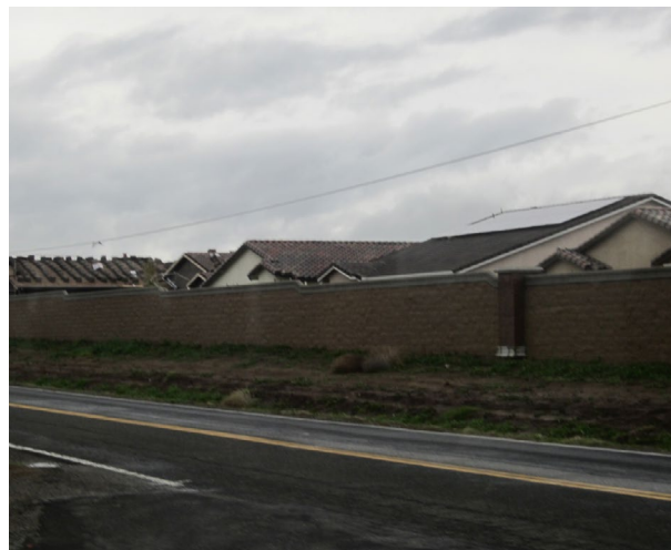
Absence of sidewalks on Church Road near Trilogy.
