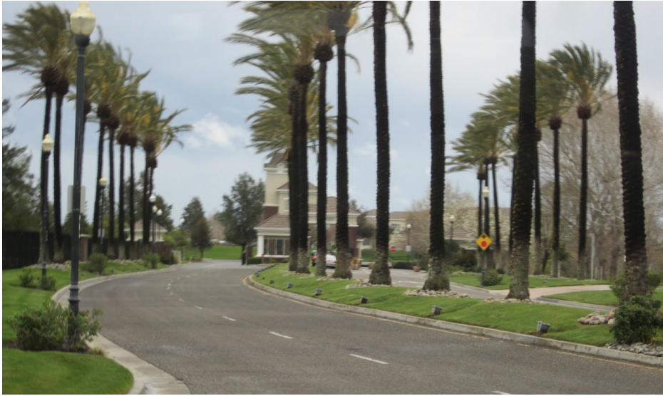
Missing sidewalks at entry to Trilogy.
