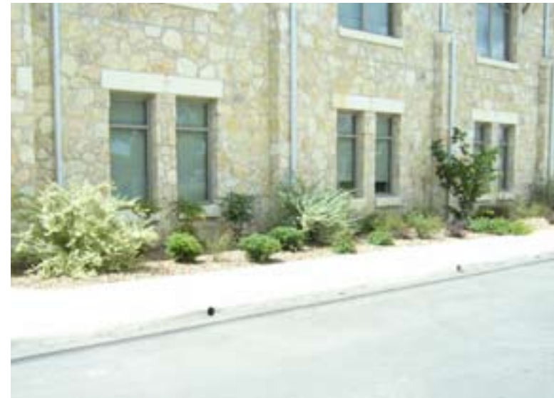
An example of missed opportunities – the storm water from this building bypasses existing planting beds and into the street and drainage pipes. These plants are probably irrigated with treated potable discharging water.
