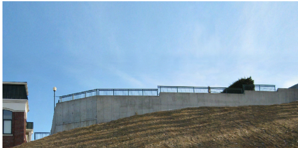
The lakeside retaining walls have a significant negative impact and can be better integrated with the local landscape with stonefacings.
