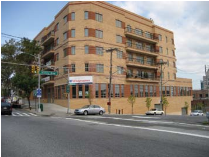
Vacant but new mixed use structures Downtown
